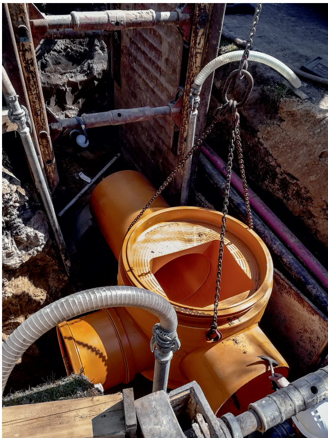
Fig. 4. Perfectly tailored to the installation environment, polymer manholes also outscore their stoneware and concrete counterparts by virtue of their lower weight © Rehau
